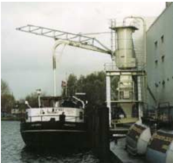
1996 : Holland - Gerkens Cacao (Gargill Group) - 1 NIV 160 tower for unloading of bulk cocoa beans with minimal breakage capacity : 150 MT/Hour
